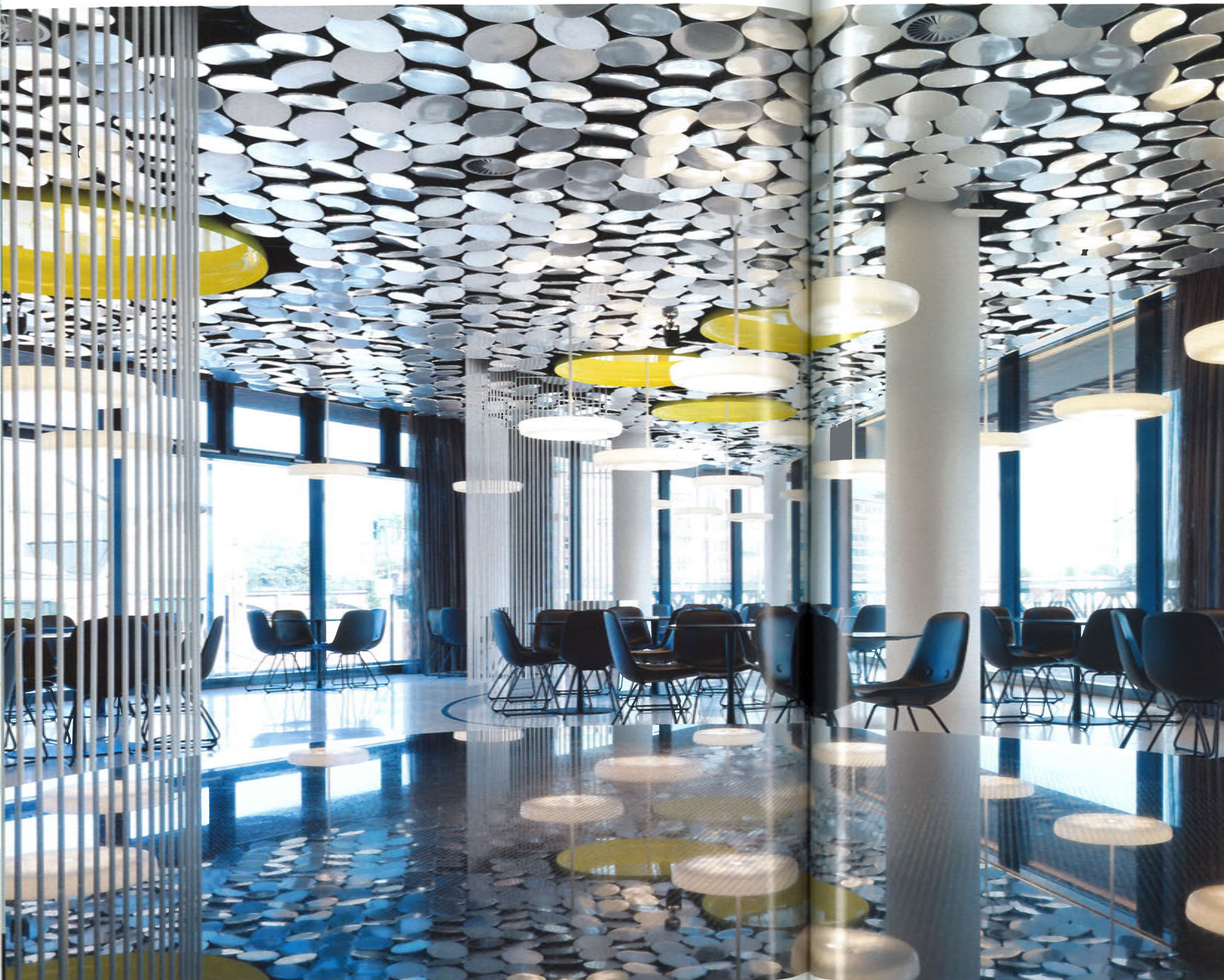
Left: Of the ceiling's 4,230 custom disks of micro-perforated satin-finished aluminum, 12 inches in diameter, 42 were modified to serve as vents. Right: Custom table bases are powder-coated steel.
