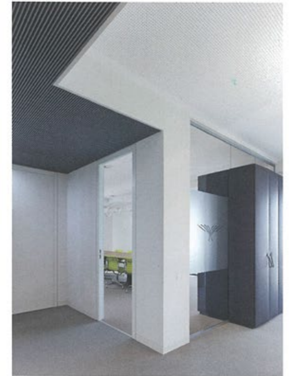
In front of the floor-to-ceiling glass walls an acoustic layer is created by positioning cupboards lined with micro-perforated artificial leather.
